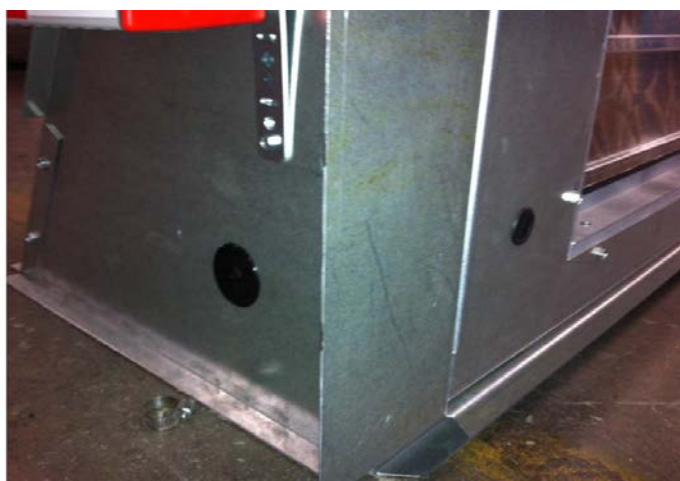
Figure 4 (Remove the bushing, cut it in one place, twist it to fit the control & power wires into it, then re-insert it into the economizer hole)
